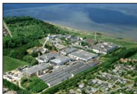
Factory in Frederikssund
